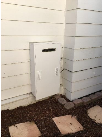
A. An exterior wall mounted tankless water heater, painted to match the adjacent wall color, with plumbing and electrical lines hidden.
