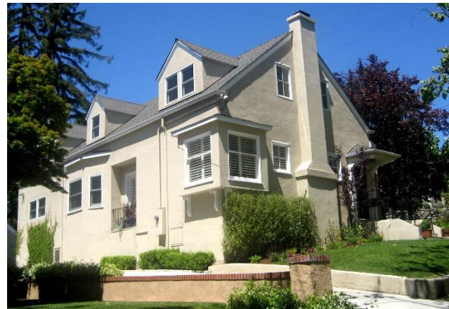
The new second floor addition uses the mix of window styles found at the existing first floor.
