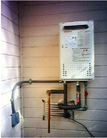
B. An exterior wall mounted tankless water heater with plumbing and electrical lines exposed.
