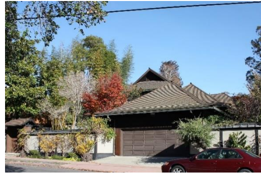
Styled Ranch-Asian: Low pitched roof with deep overhangs, exposed rafters; walls of wood and stucco.
