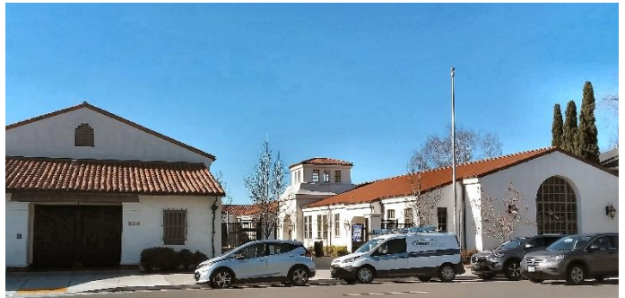
Spanish Revival – Civic: Low pitched tiled roof, little or no overhang, tower or special design element.
