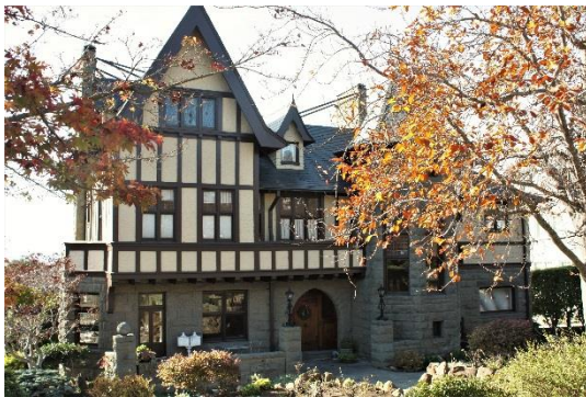
Tudor: Steeply pitched gable roofs, walls of stucco, stone and half-timbered wood.
